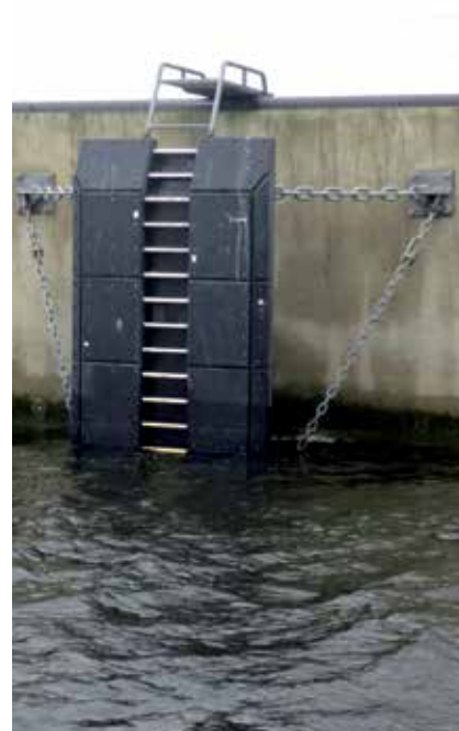
Maasvlakte II | Rotterdam | The Netherlands
