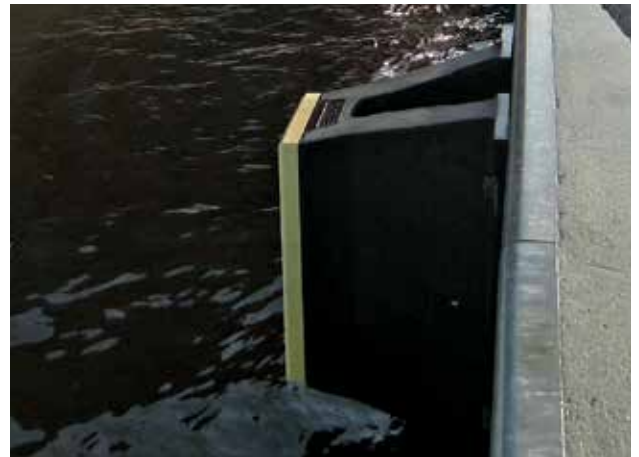
Waterland Terminal | Amsterdam | The Netherlands
