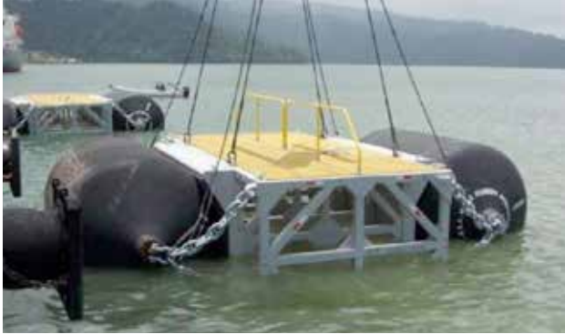
Ship Separator Installation | Guatemala
