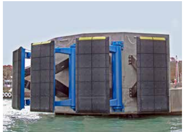
Ferry Terminal | Gotland Island | Sweden
