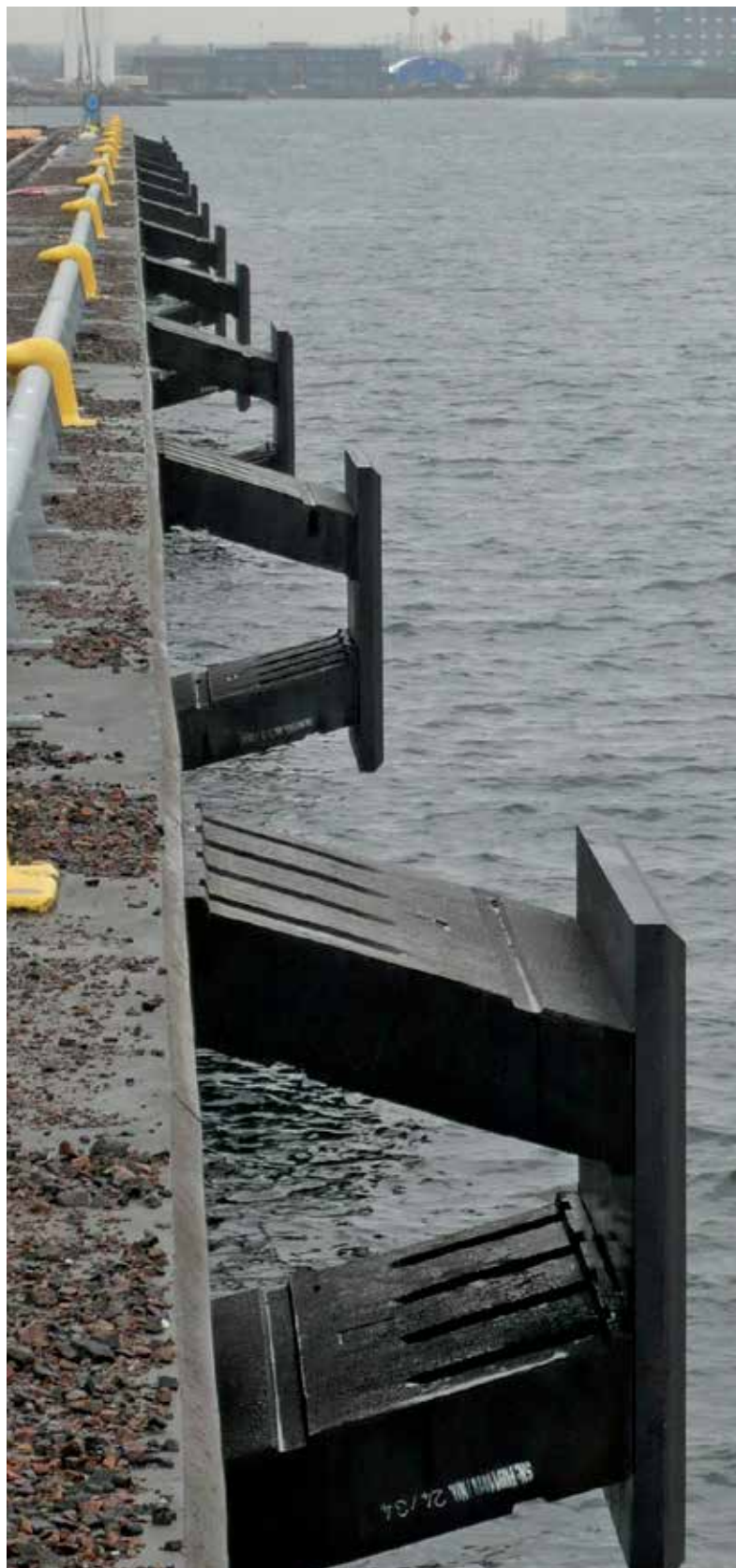
Ferry & RoRo Terminal | Malmö | Sweden
