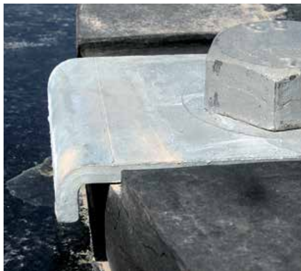
Maasvlakte II | Rotterdam | The Netherlands
