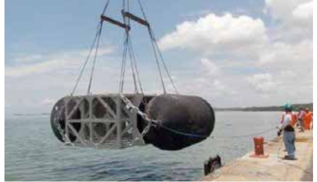
Ship Separator Installation | Guatemala
