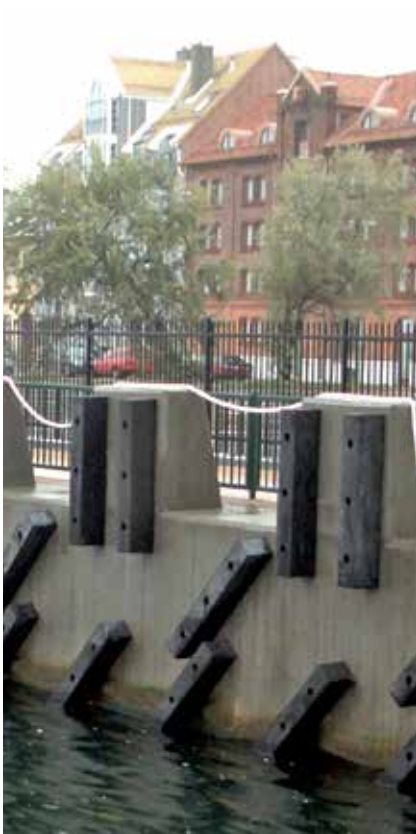
Ferry Terminal | Landskrona | Sweden
