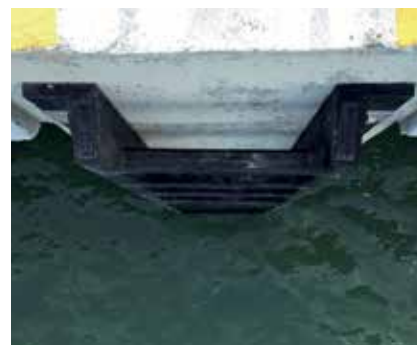
Feed Solid Product Jetty | Johor | Malaysia
