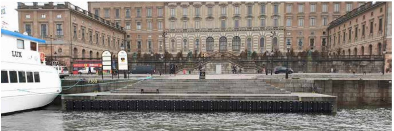
Logårdstrappan | Stockholm | Sweden
