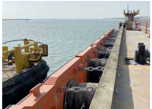
RoRo Facility | Portland, TX | USA
