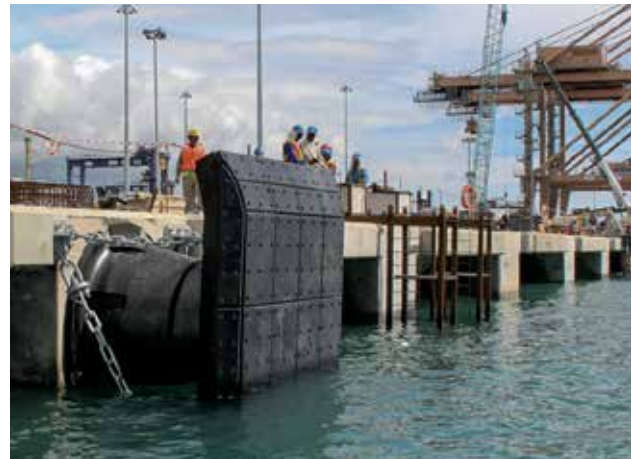
Mauritius Container Terminal | Port Louis | Mauritius
