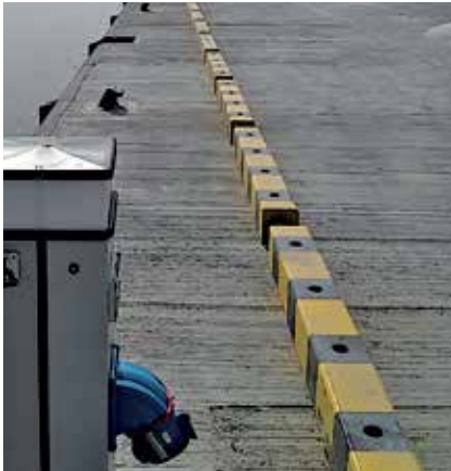
Southern Quay Wall | Simaisma | Qatar
