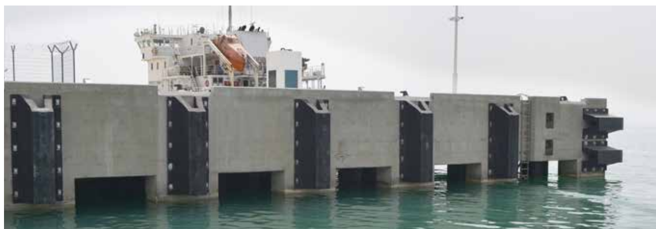
Turkmenbashi International Seaport | Turkmenbashi | Turkmenistan
