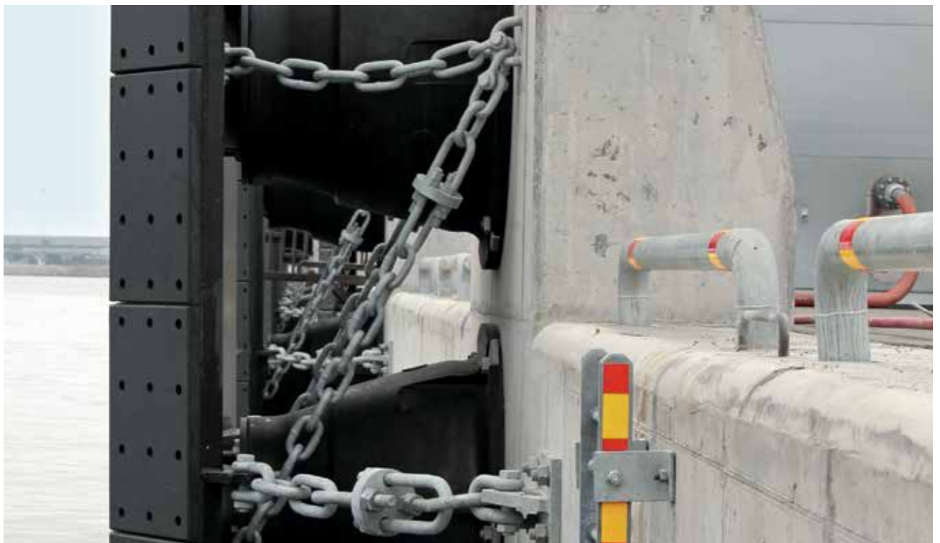
Restraint chain assemblies and brackets
