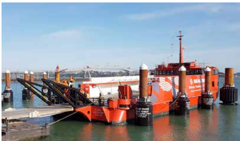
SeaLink Terminal | Auckland | New Zealand
