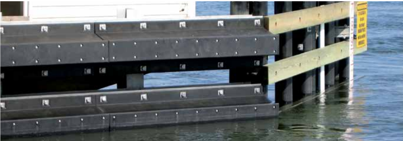
Margate Bridge | Margate City, NJ | USA
